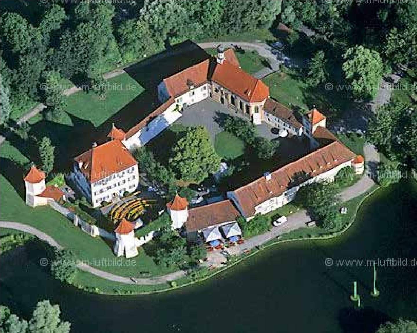
SCHLOSS BLUTENBURG RENOVATION | MUNICH
