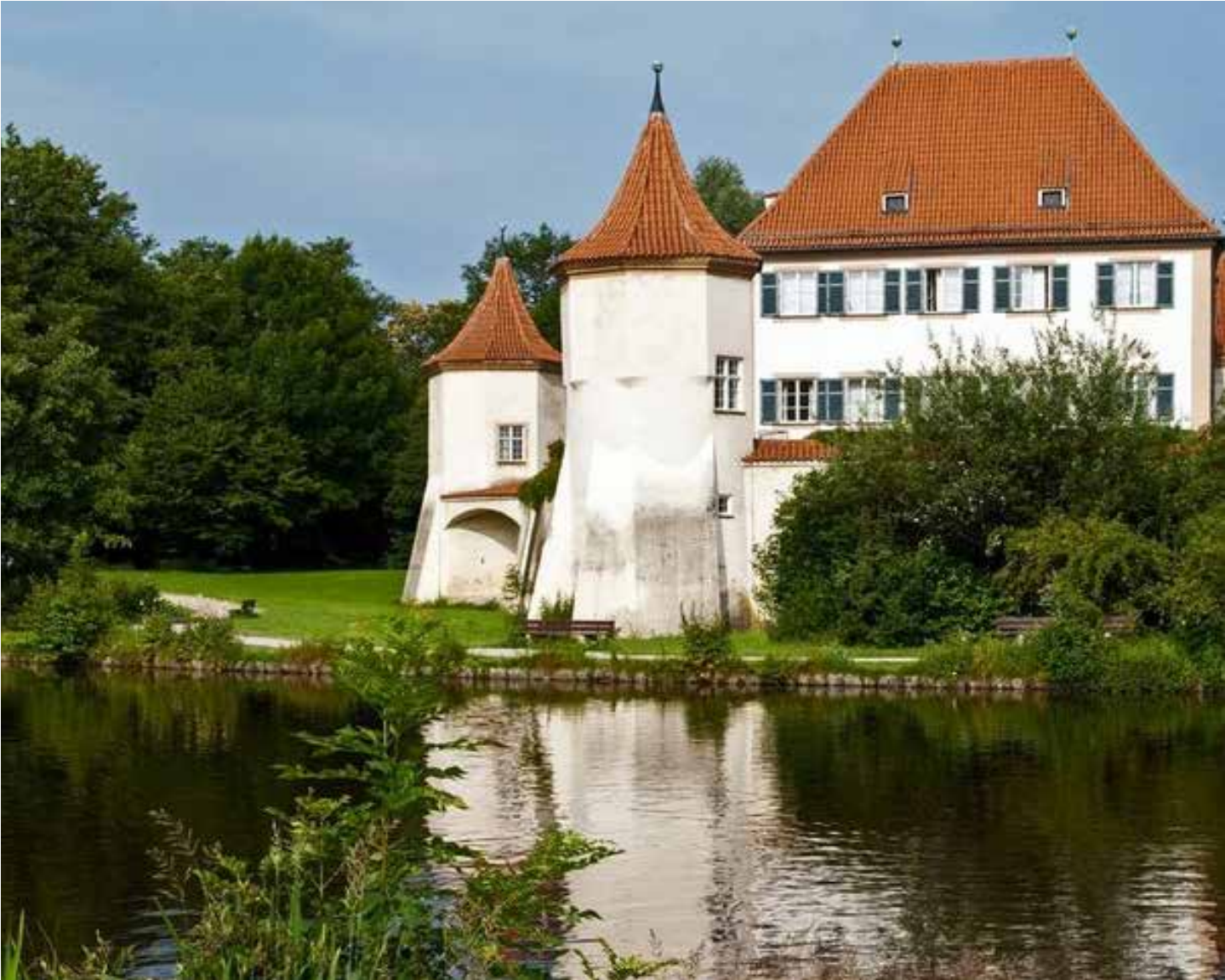
SCHLOSS BLUTENBURG RENOVATION | MUNICH
